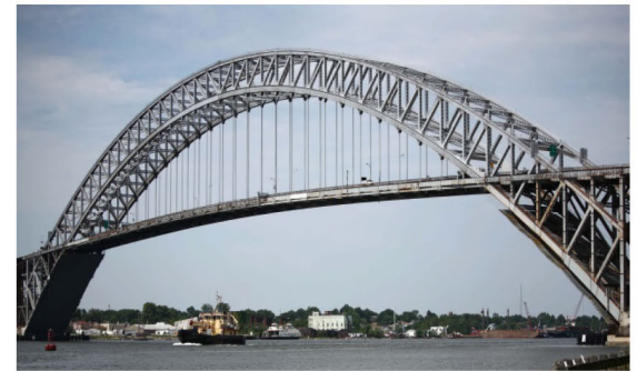
Arches support their loads in compression
