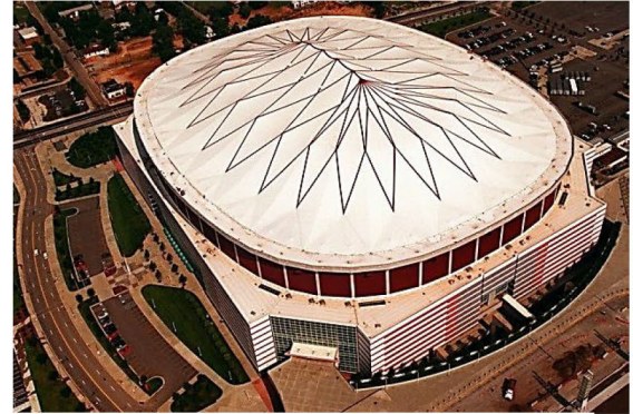
The roof of the “Georgia Dome” in Atlanta, Georgia can be considered as a thin membrane.
