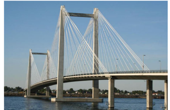
Cables support their loads in tension.
