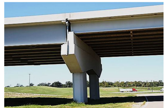
The prestressed concrete girders are simply supported
